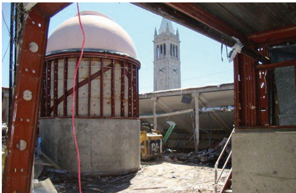
Former dome before demolition.
