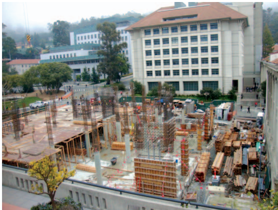
New Campbell hall rising.
